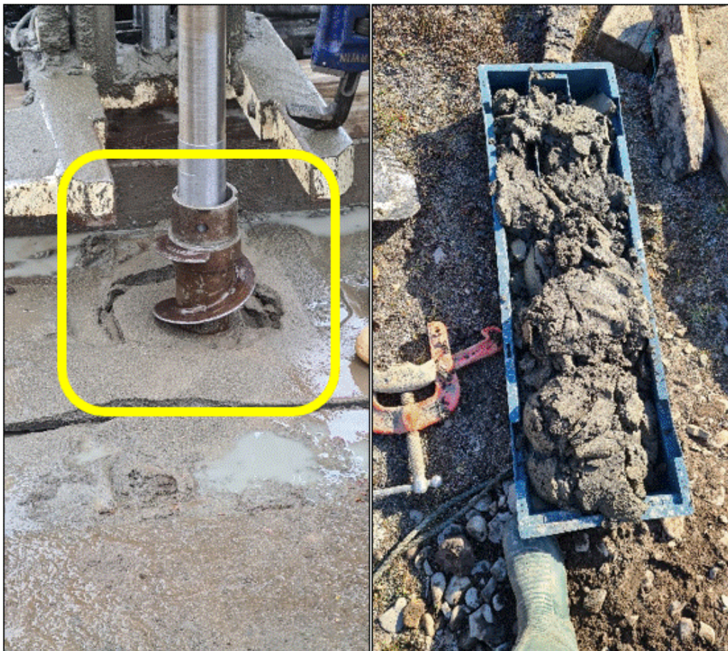
Figure 4: Sand reject material being ejected from hole (left), collected/sampled sand reject material (right)
