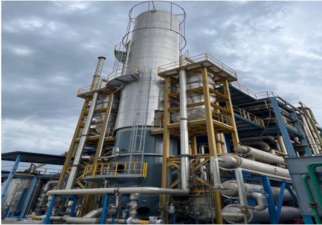
oil storage and extraction facility Figure 3. Partial view of biofuel plant including distillation column
